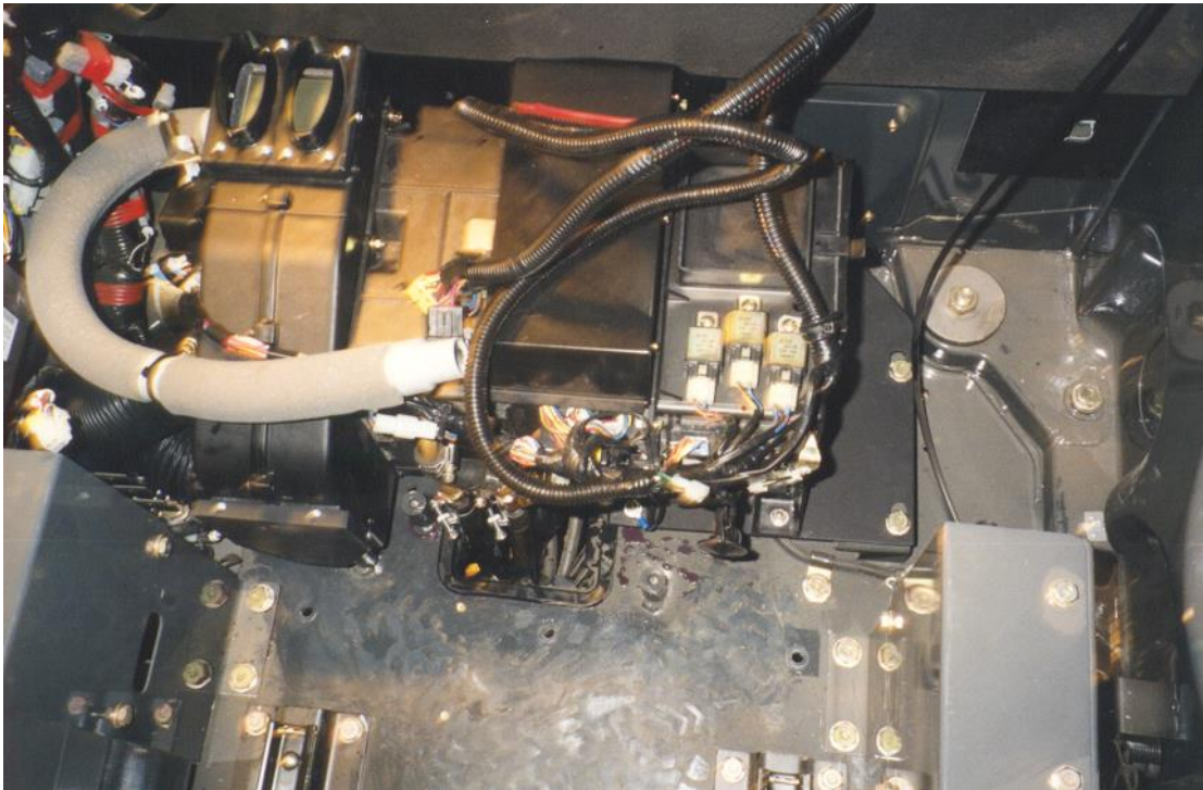
Evaporator assembly mounted in place.
